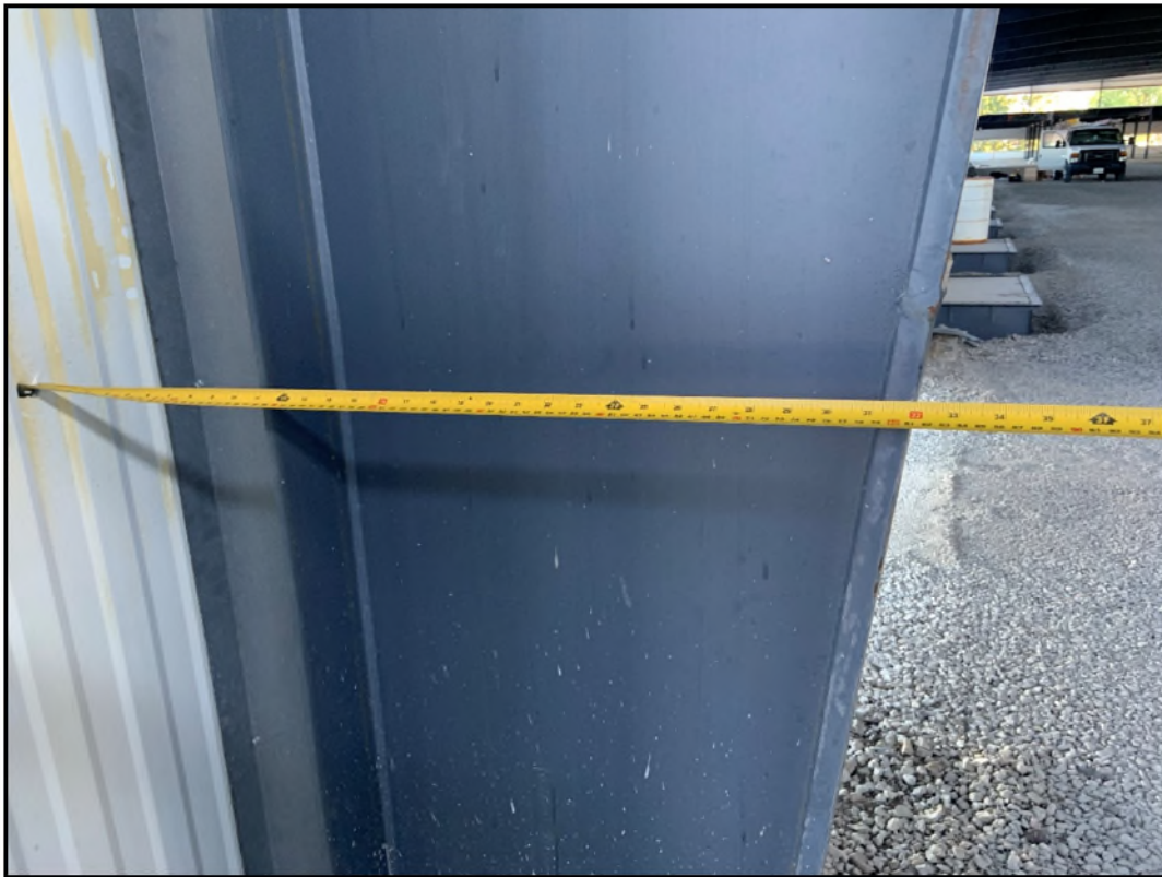
32" depth of wall space at 48" high, from the inside of the IMP to the inside of the load bearing post
