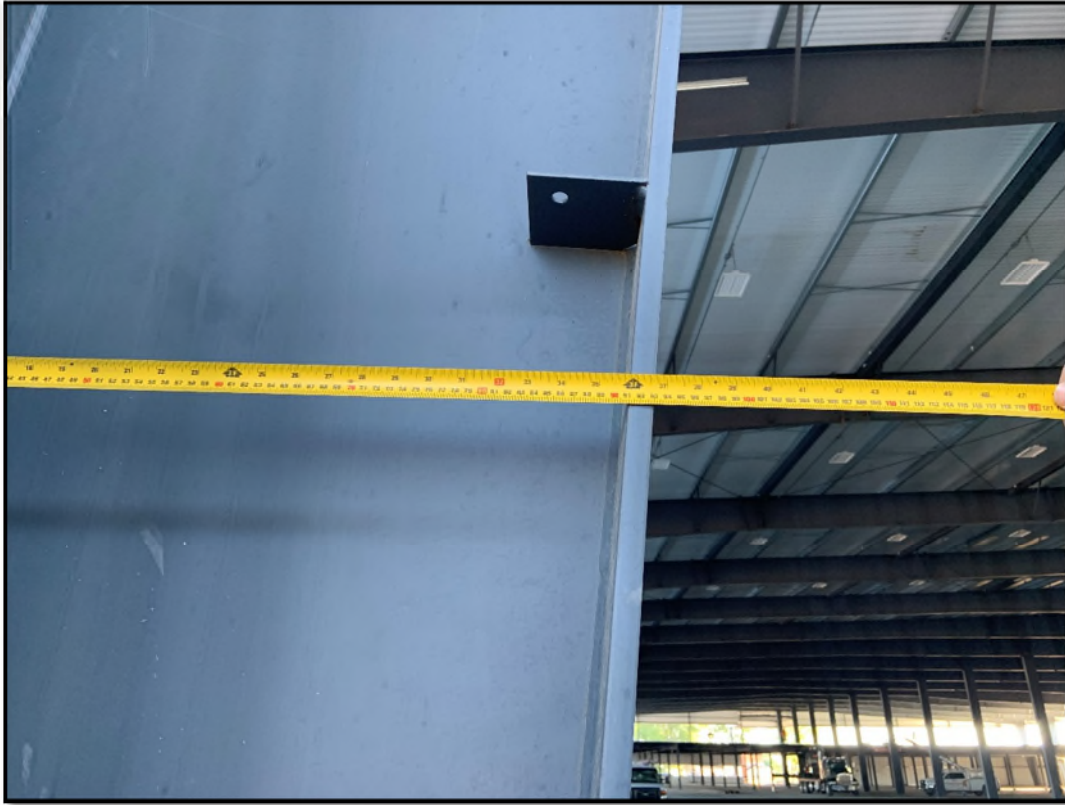
36" depth of wall space at 84" high, from the inside of the IMP to the inside of the load bearing post
