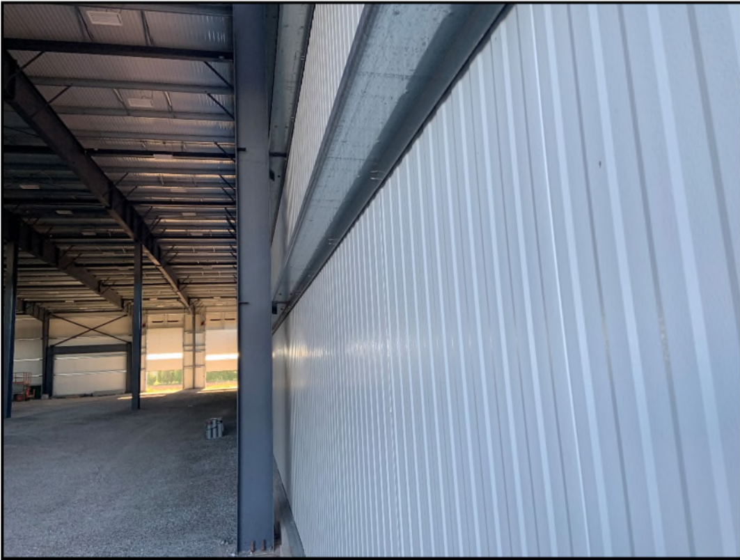
Interior view of gable end with Insulated Metal panels used on a warehouse
