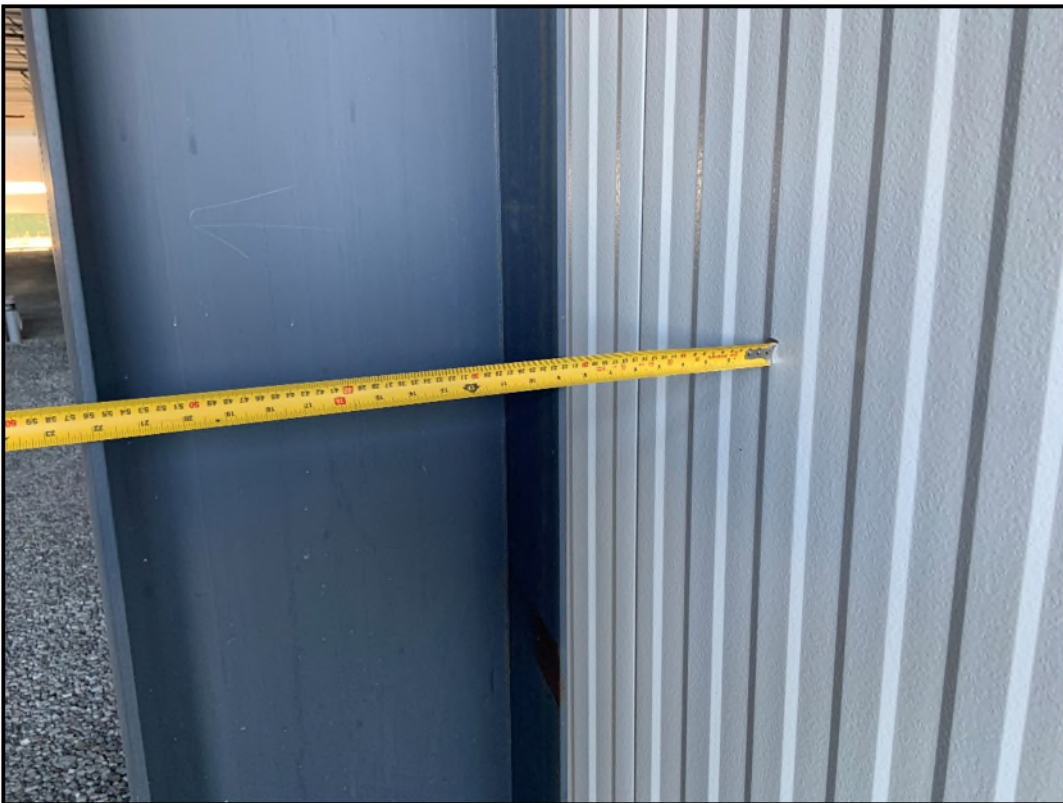
22" depth of wall space from the inside of the IMP to the inside of the narrow gable post.
