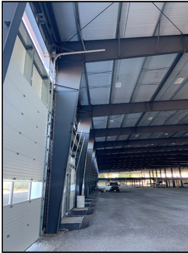
Interior view of load bearing wall with Insulated Metal Panels used on a warehouse
