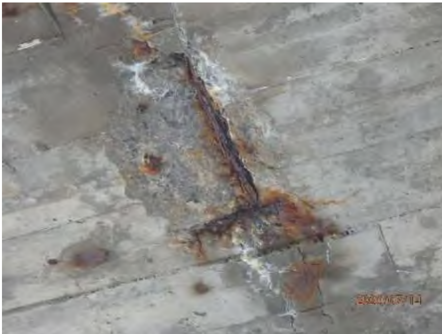
Photograph No. 4: 0174: Spall near mid span.
