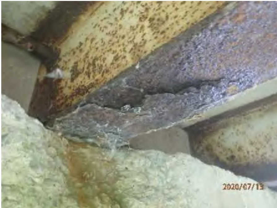
Photograph No. 4: 0172: Severe corrosion with loss of cross section area and loss of bearing seat at northwest corner.
