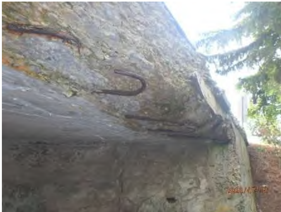
Photograph No. 4: 0116: Exposed corroded reinforcing steel at west end.
