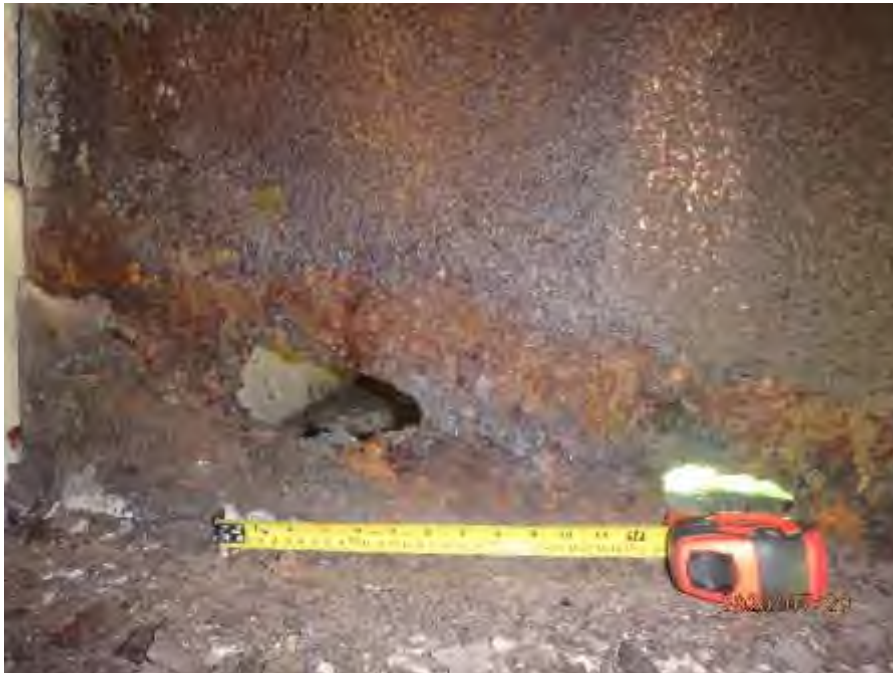
Photograph No. 4: 0082: Perforations at the south end of the east exterior girder.
