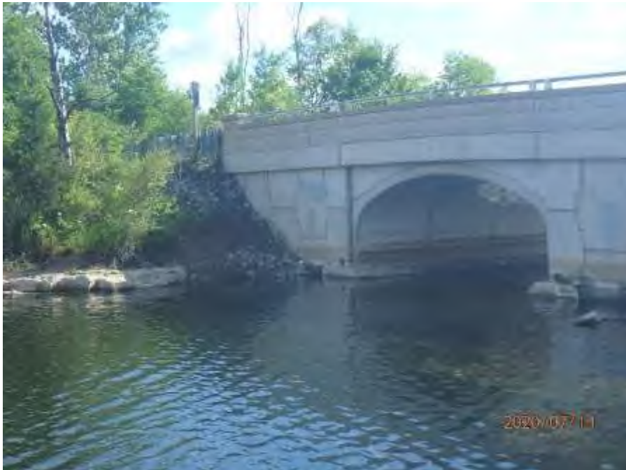
Photograph No. 4: 0038: Erosion at the northwest corner.
