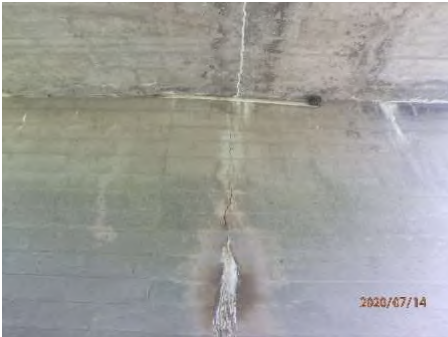
Photograph No. 4: 0328: Crack in bridge deck soffit and abutment sidewall.
