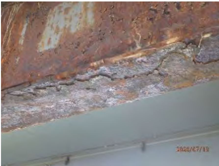
Photograph No. 3: 0305: Medium to severe corrosion of center girder, at north end.
