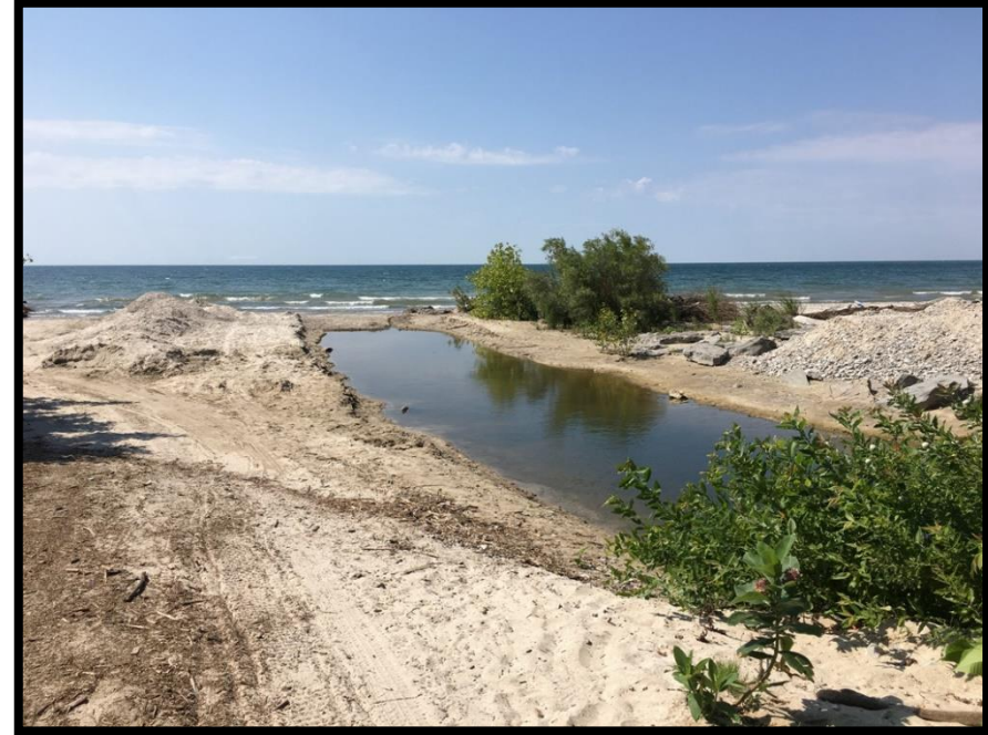
8.1.17 – Outlet obstructed with Sand
