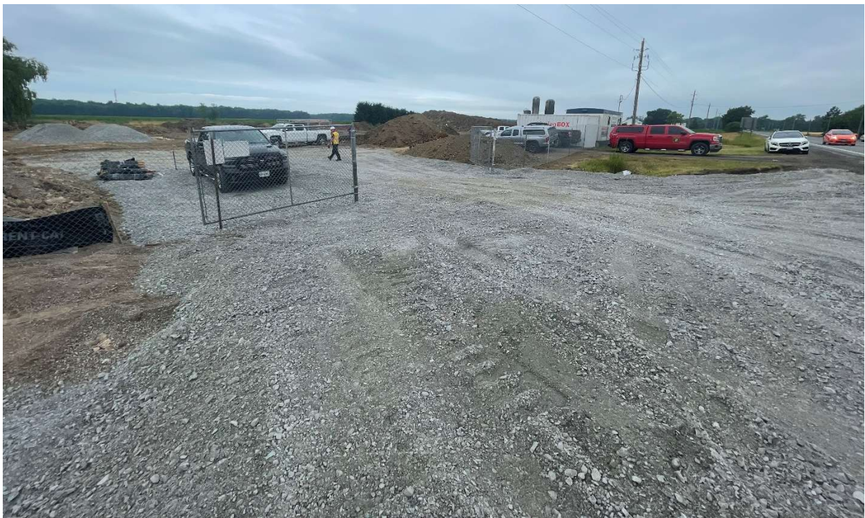
New Site Entrance Constructed
