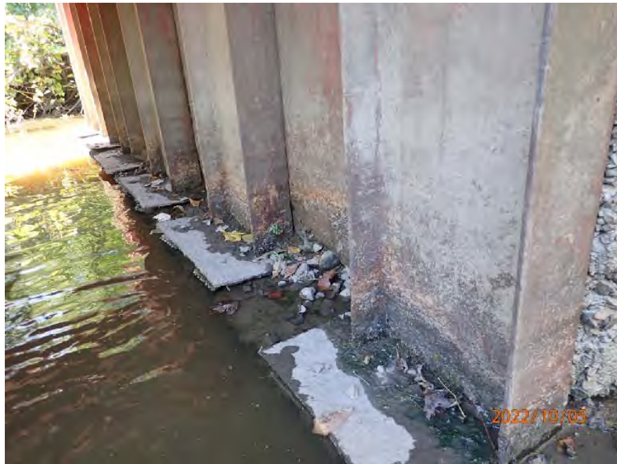
Photograph No. 4: 0446: Corrosion in vertical steel base plates (typical).
