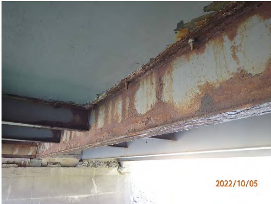
Photograph No. 4: 0487: Severe corrosion of center girder (typical).
