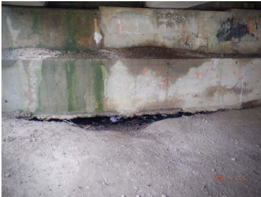
Photograph No. 4: 4828: Large void under north abutment.
