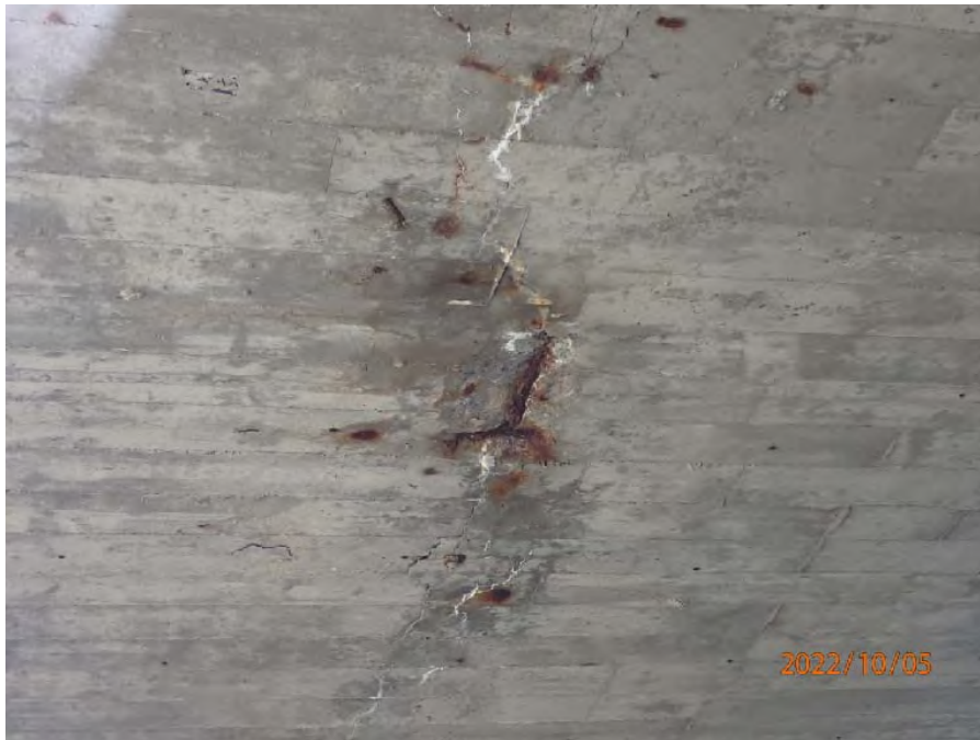
Photograph No. 4: 0229: Spall near mid span.
