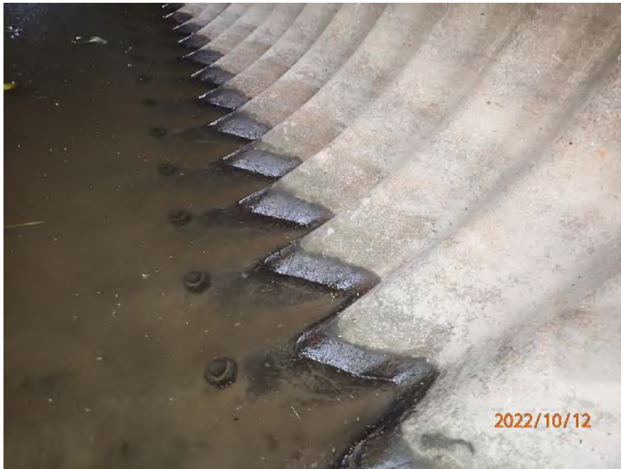
Photograph No. 4: 0146: Corrosion at waterline (typical).
