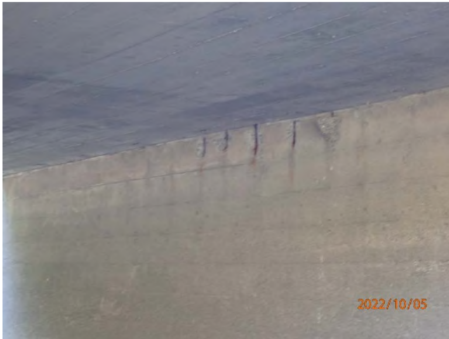
Photograph No. 4: 0108: Spalling in south abutment.
