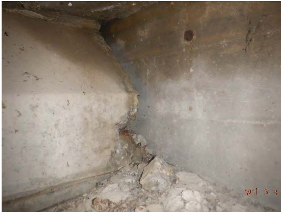
Photograph No. 4: 6448: Deterioration at the end of the girder (typ).
