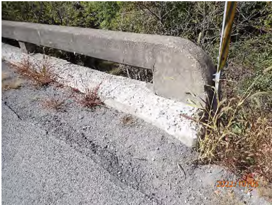
Photograph No. 4: 0264: Disintegration of west concrete curb.
