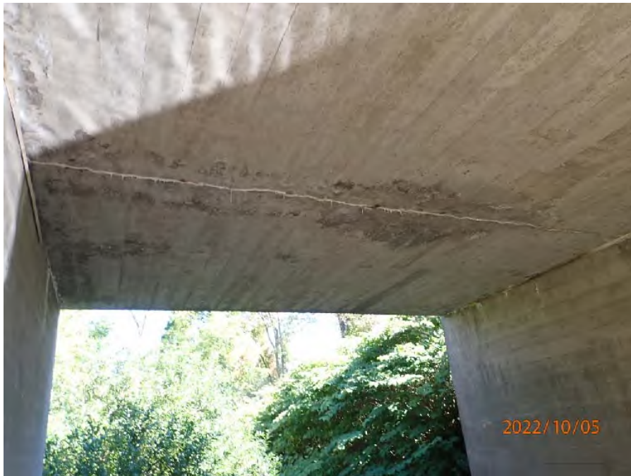
Photograph No. 4: 0255: Crack in bridge deck soffit.
