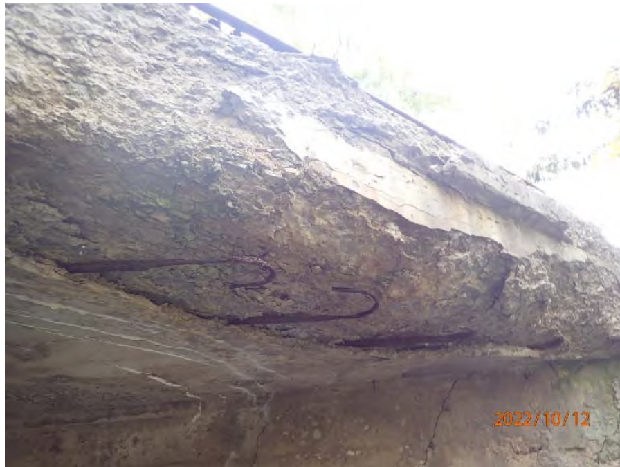
Photograph No. 4: 0112: Exposed corroded reinforcing steel at west end.
