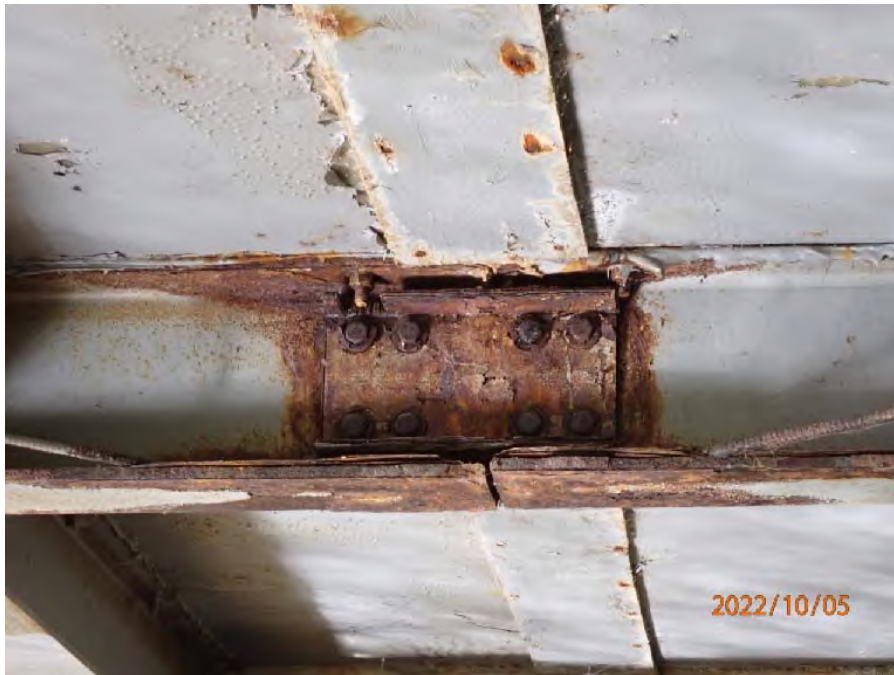
Photograph No. 4: 0349: Corrosion in steel work at centre of structure.
