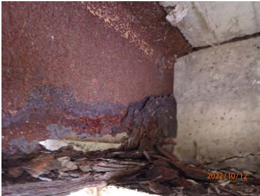
Photograph No. 4: 0062: Severe corrosion and perforation at second girder from the east on the south side.
